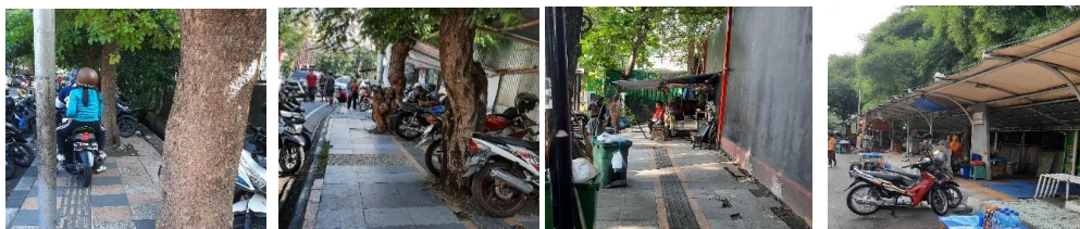
Gambar 6. Hambatan Pedestrian Jalan Pandanaran II
