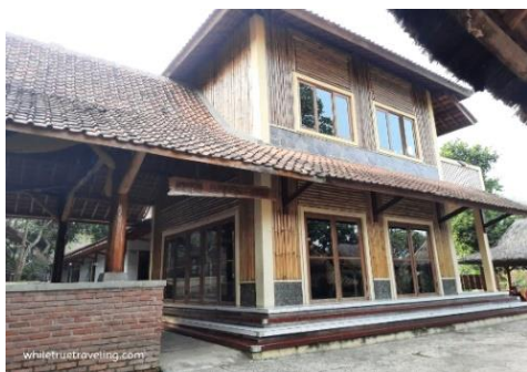
Figure 2. Façade of Bale Sarasehan
