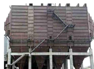
Fig. 13. Pulse Jet Bag Filter
