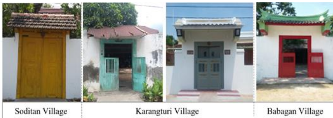
Fig. 5. The Peranakan Houses in Three Pecinan, Lasem
