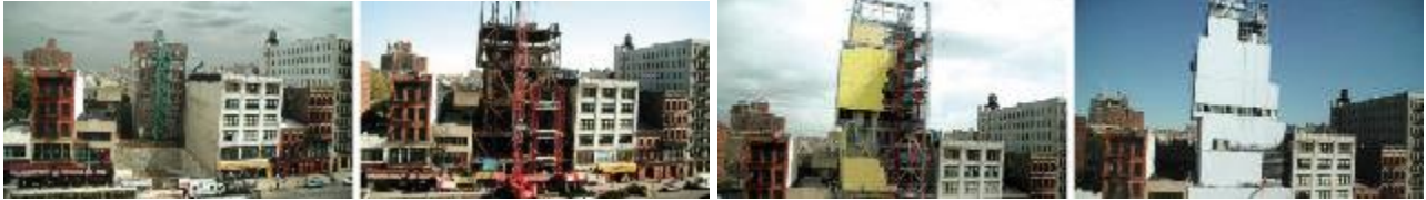
Gambar 2. The New Museum Sumber: https://www.newmuseum.org/building
