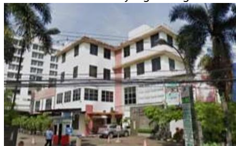
Gambar 10. Kondisi fasad Malibu Dome Convention Hall
