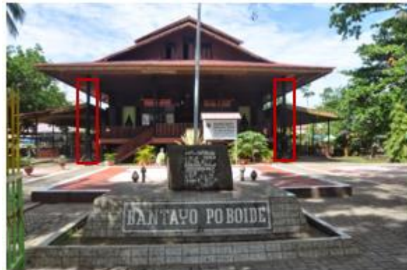
Figure 1 The main pole or Wolihi that stuck from the ground directly into the roof truss
