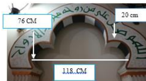
Figure 5. Archway in the women's prayer room Hunto Sultan Amay Gorontalo Mosque (Source: researcher personal documentation, 2018)
